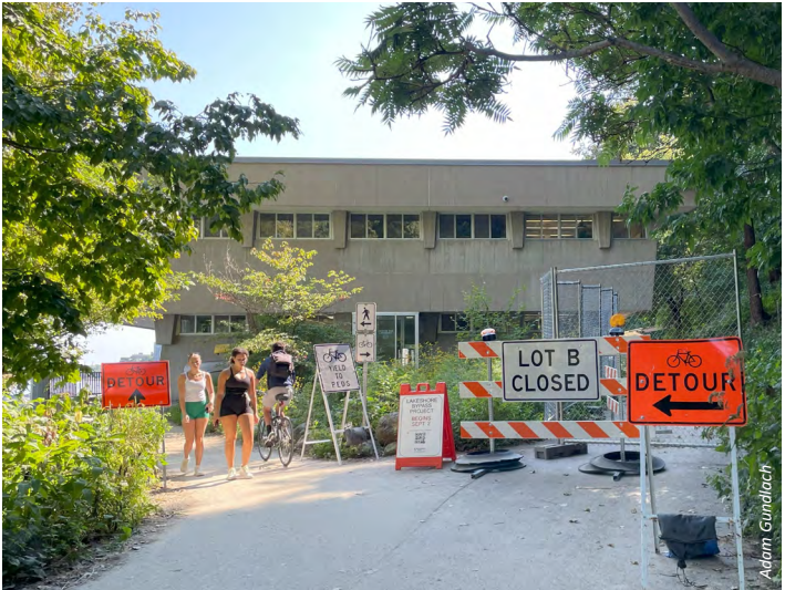
Work on the Temin Lakeshore Path at the Limnology Building has begun and is expected to last through November. The path south of the building is being reconstructed to improve safety for users.
